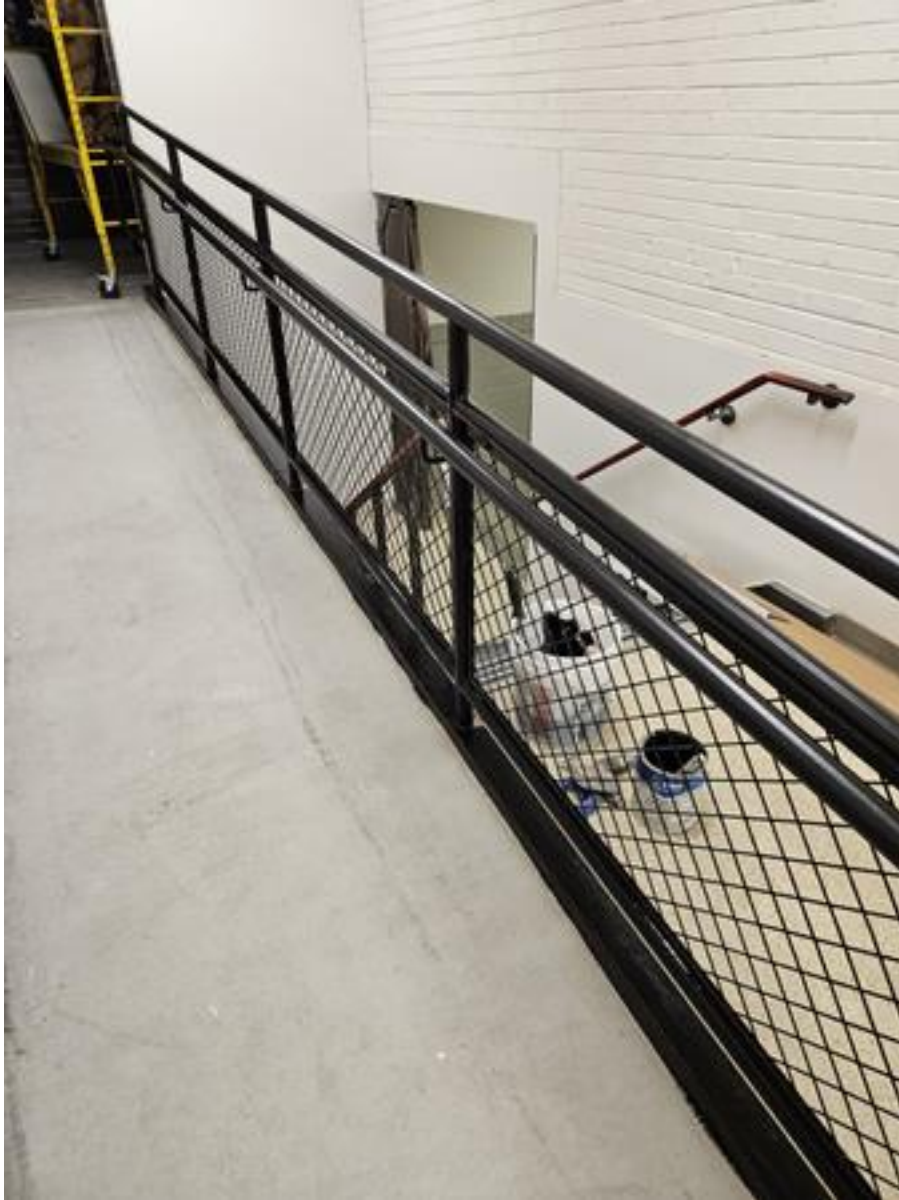
Painting the Ramp Handrail
